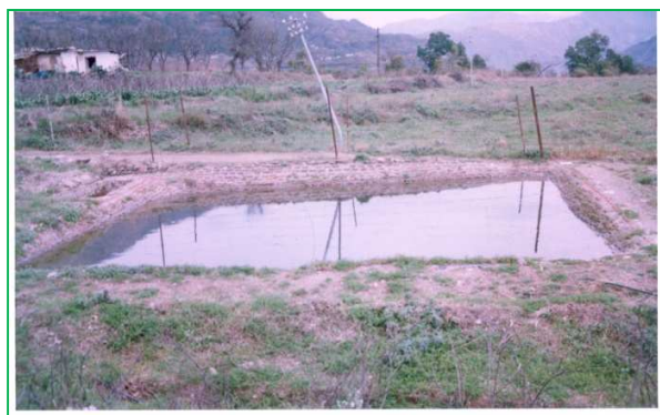
Fig. 5: poly lined farm pond with brick pitching
