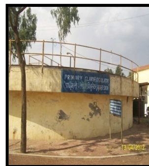
Figure 2b :Primary clariflocculator
