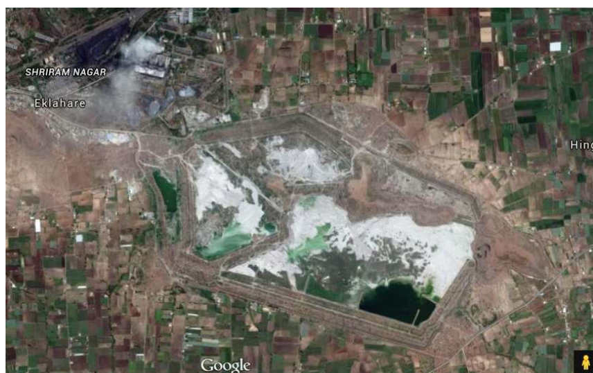
Image 1: Showing the Eklahare Thermal Power Plant and Fly ash Dumping Ground
