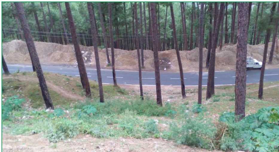
Fig.7: Mobilized material of building construction (mismanaged)-Karbala
