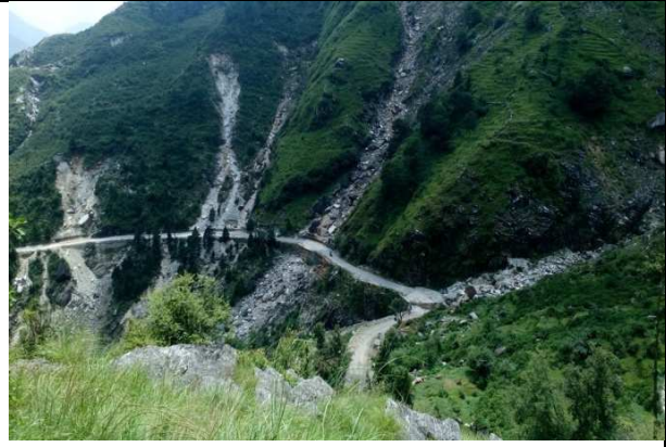
Fig. 3: Debris Channel Flow In Jhekla Village
